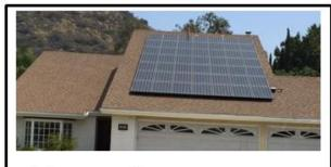
Retro-fit job. Distracting high-contrast silver over black cells. Front-facing. Does not lay flush with the roof. Too much glare.
